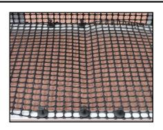
**23)** Insert Push Rivets through mesh into pre drilled holes.
